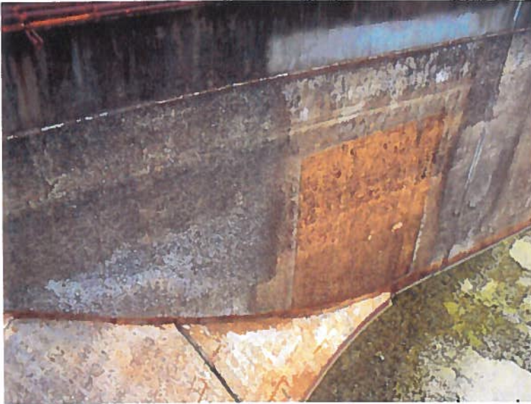
Overview of Carboline panel (P-10) 510 SG/Fiber Reinforced PolyBrid 705.
