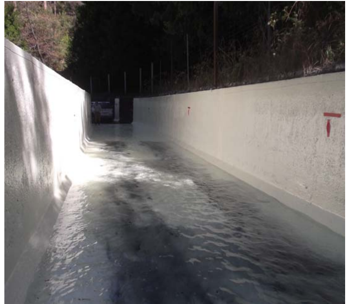
Figure#4: Overview of Adhesion Test Location Station 337+36.
