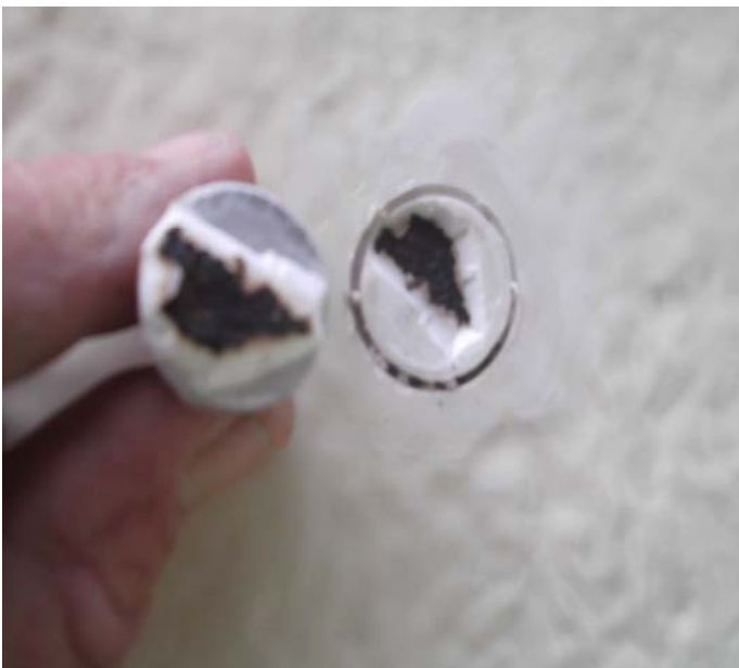
Figure#3: Site #6 Scored Dolly, 750 PSI Coating Failure.
